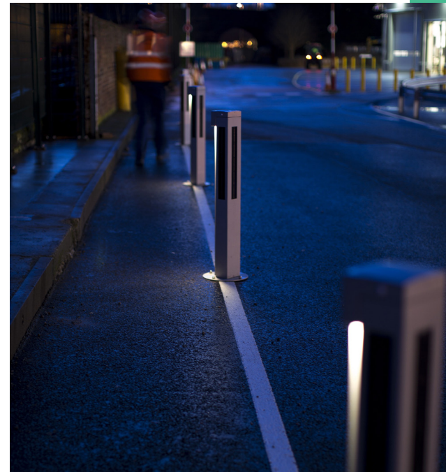
The revolution in small solar batteries has created an off-the-grid vocabulary for trail lighting. Solar LED is an example. A solar-powered LED delineator is used for bike lanes, walking, and hiking trails.
